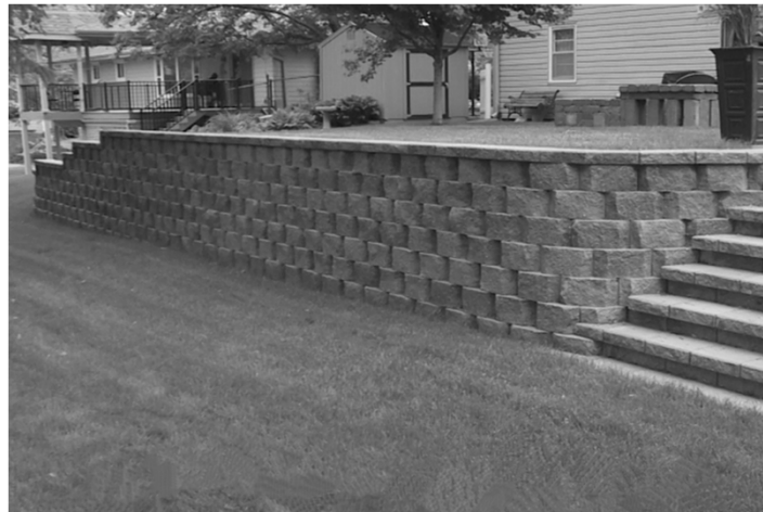
Not cited – Not in normal path of travel (Retaining Wall)
